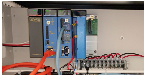
Figure 2: Photograph of the newly installed PLC subsystem for the irradiation in the patient-monitoring room. From left to right, power supply, sequence CPU, Linux CPU, and digital input modules, respectively.
