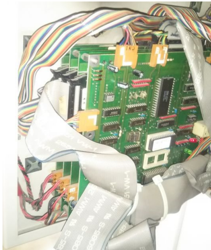
Figure 5: Photograph of personnel key system control board.
