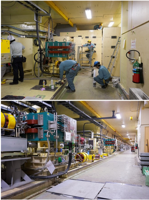
Figure 3: Picture of before (top) and after (down) integration of Linac.
