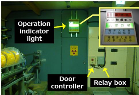
Figure 7: Picture of the operation indicator light and the door controller attached to shield wall before removal at the dividing point of Linac.
