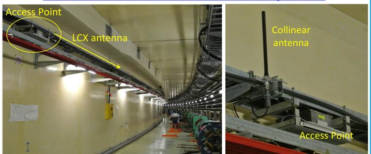
We select LCX and Collinear antennas with good radiation hardness >1MGy.
