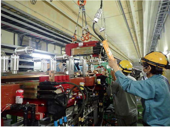
Wiggler magnet disassembly
