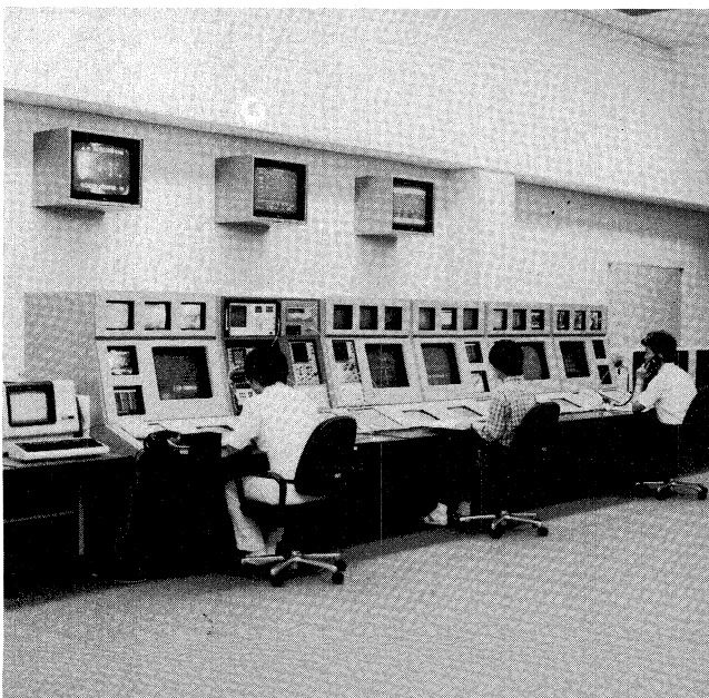
Fig. 4. One day, a view of the control room.
