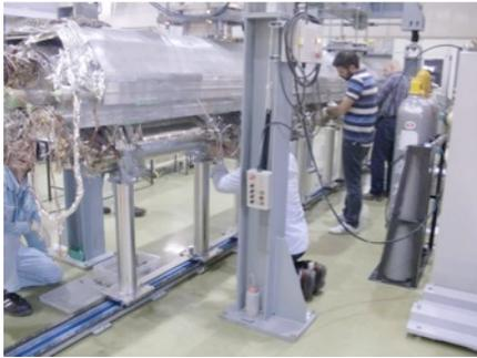
Fig. 2: Dis-assembly of S1-Global cryomodule by INFN and FNAL team.
