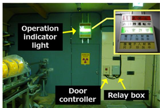
Figure 8: Picture of the operation status indicator and the door controller at the shield wall before removal at the dividing point of Linac.
