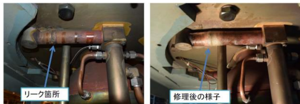
Figure 1: Location of the water leak on the cooling pipe at the klystron installed to D11-C.
