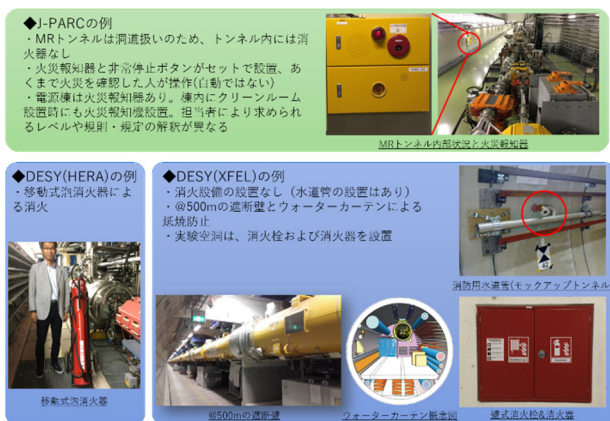
Figure 17: Fire protection in J-PARC and DESY.
