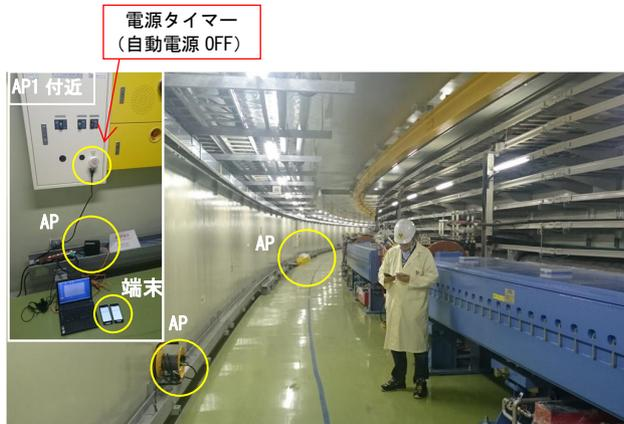
Figure 4: Positioning sensor network system in MR tunnel.
