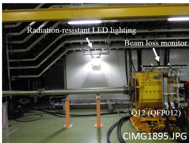
Figure 1: Setup of the Radiation-resistant LED lighting.
