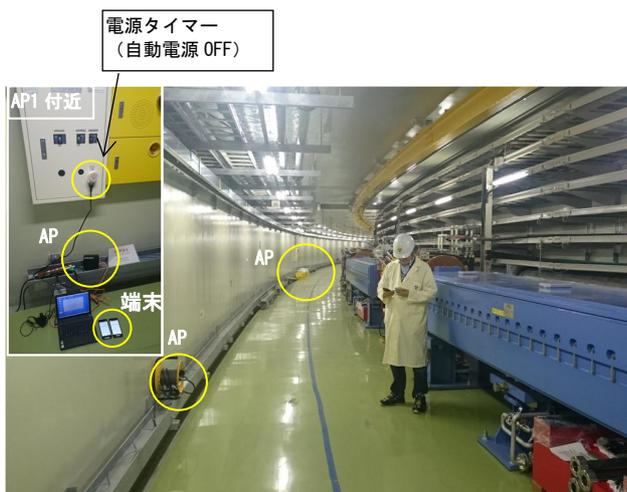
Figure 5: Positioning sensor network system in MR tunnel.
