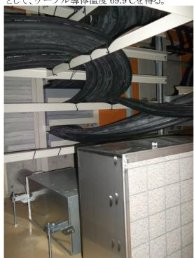
Figure 4: Cable cooling system with FDF.
