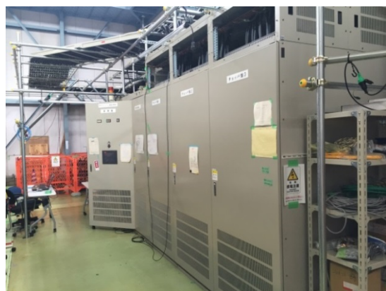
Figure 3: Test power supply(Old PBH1).
