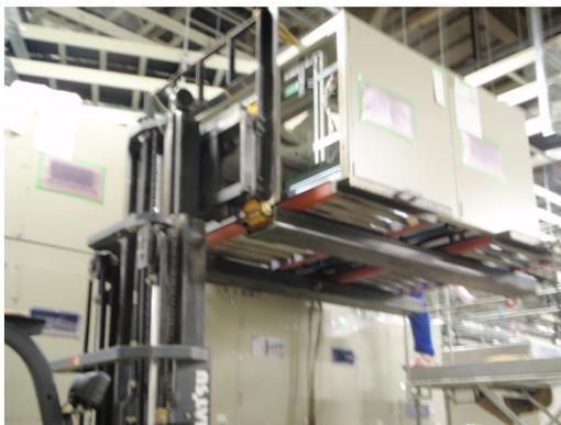
Figure 8: Installation work of a cabinet of added inverter units.
