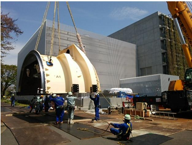
Figure 8: Installation of the gantry structure to the gantry room in NIRS.
