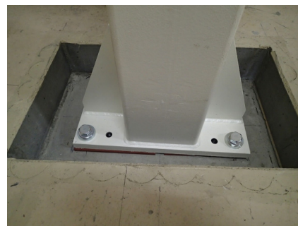
Figure 4: Column base plate
