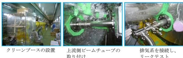
Figure 13: Installation of a beam tube at upstream side.
