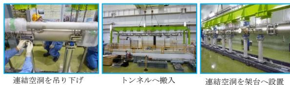
Figure 8: Transportation of stringed four cavities into the STF tunnel.
