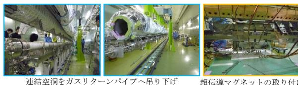
Figure 10: Hanging of eight SC cavities under GRP (gas return pipe) and installation of a SC magnet.
