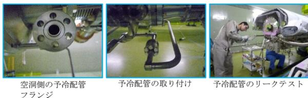
Figure 11: Connection of pre-cooling pipes.
