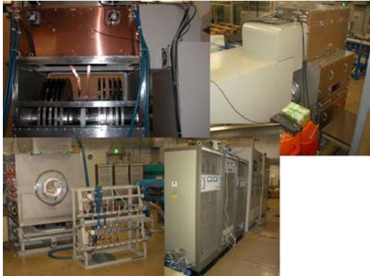
Figure 4: A prototype of RF system in the RCNP, Osaka University.
