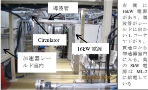
Figure 2: Waveguide of ML
